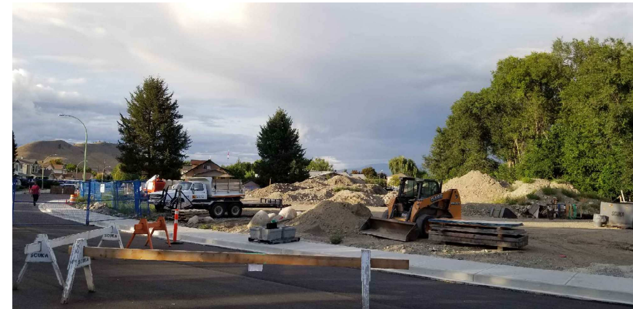
4 PHOTO 2 (2019) VIEW LOOKING NORTH TO SITE
